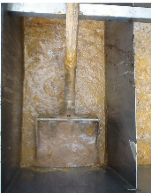
A large amount of food debris scooped from bottom of the trap.
