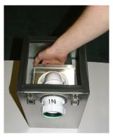
4. Slide bracket & filter until clear of inlet pipe.
